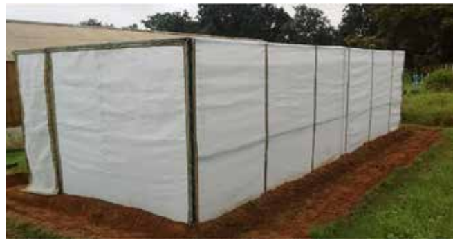
Fig. 117: Insect proof net house fabricated for the study
