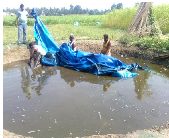
Fig.9 Removal of silpaulin/polyethylene sheet from the pond and cleaning in the micro-pond
