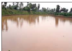
Water storage in De-silted pond
