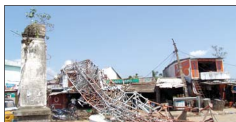
Infrastructure damage in Hudhud
