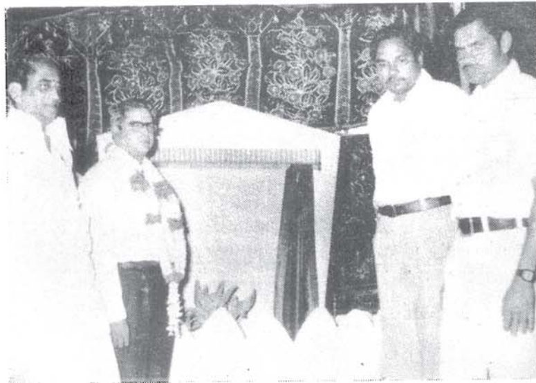
The foundation stone for residential complex for the staff of CTRI Research Station, Kandukuru was laid on 10th August, 1982 by Dr. N. C. Gopalachari, Director.
