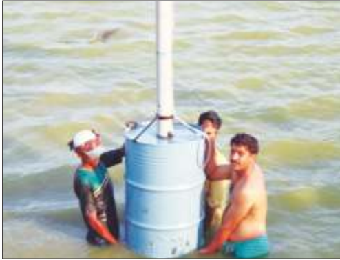
Installation of seepage measurement device
