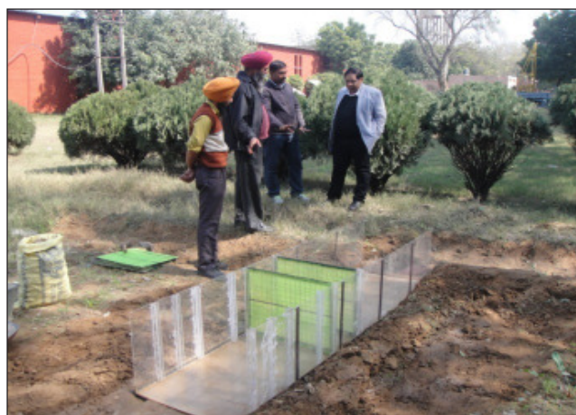
Plate 3.2.1. Fabrication and installation of composite filter in the field
