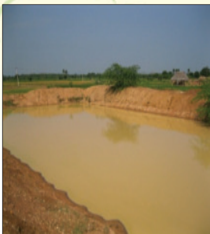
Construction of rainwater harvesting structure
