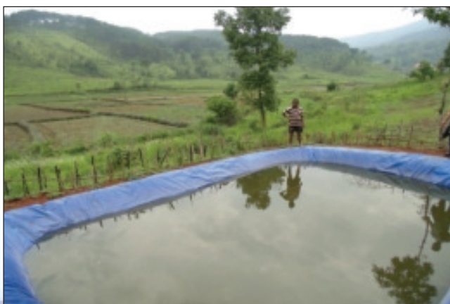
Plate 2.11.2. Jalkund at Mawpun village
