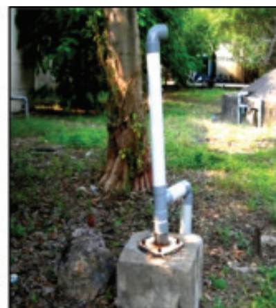
Fig. 3.1.4. Auto distribution system for roof water runoff
