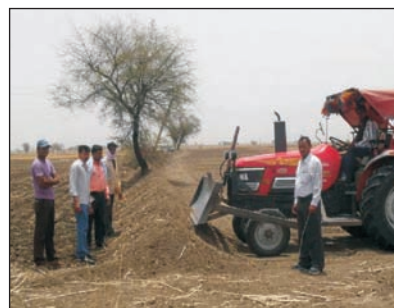
Field bunding for in-situ moisture conservation
