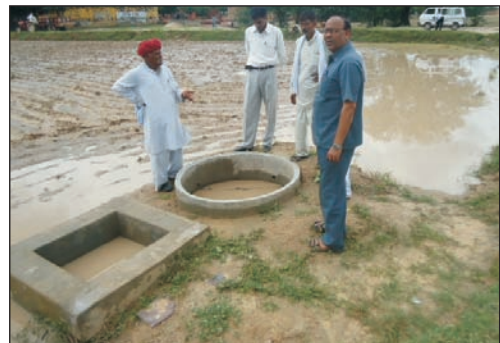
Tube well recharging
