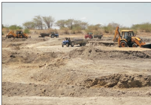
Pond de-silting in progress
