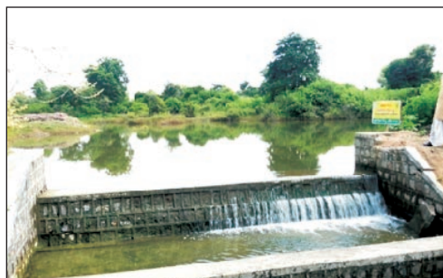
Renovated check dam
