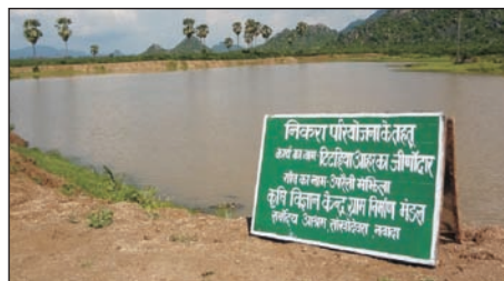
Renovated water reservoir
