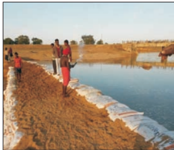
Construction of sandbags check dam by villagers
