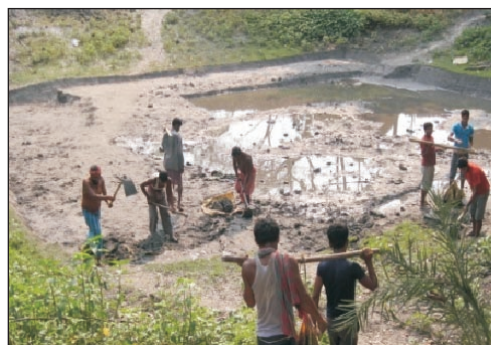
Pond renovation work in progress
