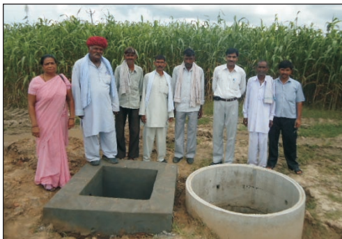
Constructed tube well
