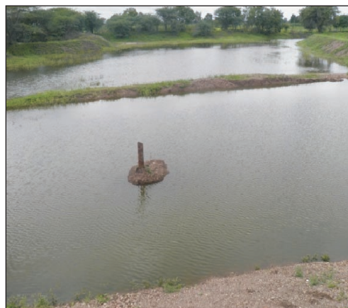
Water storage tanks after de-silting
