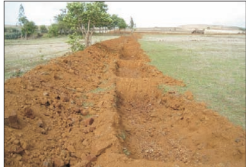
Trench cum bunds dug across barren lands
