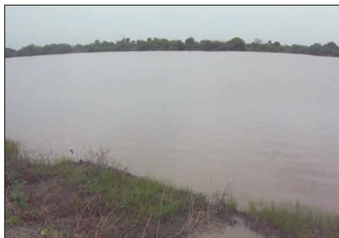
De-silted pond filled with water
