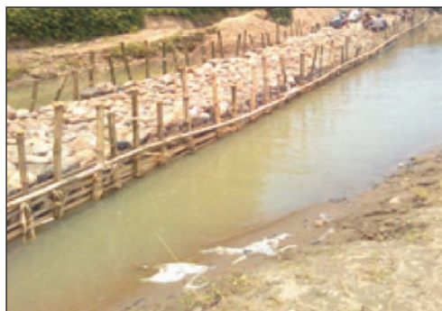
Rock filled dam constructed by villagers
