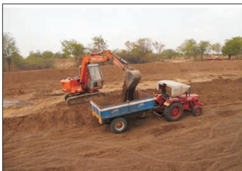
De-silting in progress
