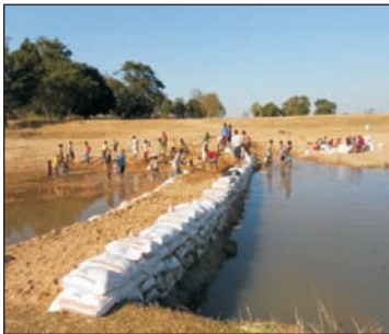
Construction of sandbags check dam by villagers
