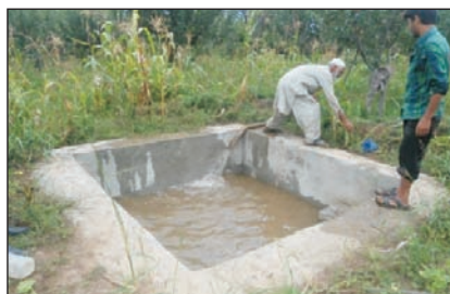
Improved water storage structure
