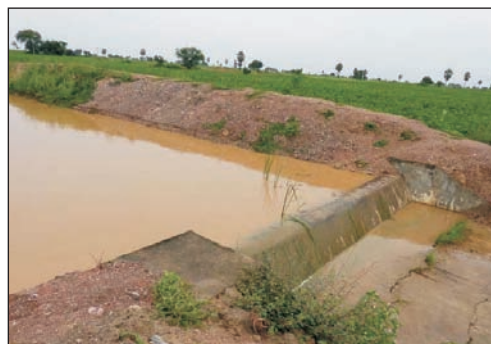
Newly constructed check dam
