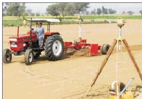
Laser leveling in progress
