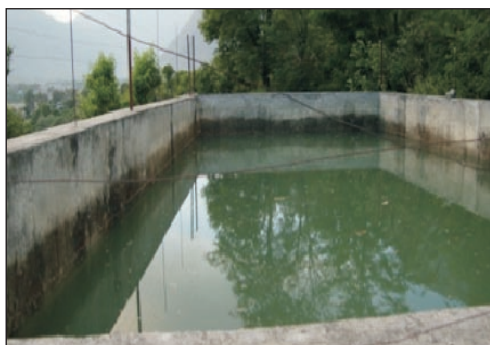
Renovated water storage tank
