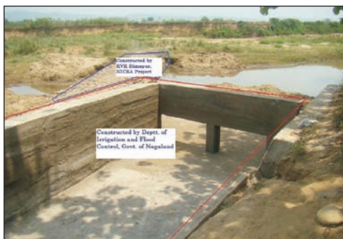
Rock filled dam and the irrigation channel constructed under NICRA
