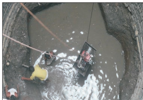
De-silting of open well in progress
