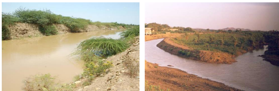
Rejuvenation of Ichalahall stream
