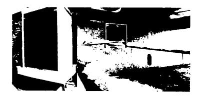
intricately woven cellulose pads provide necessary water to air contact to achieve high efficiency in cooling. The feeding side and the entrance side of the shelter have been covered with net and tarpaulin to prevent solar radiation input and the cold air from escaping the shelter.
