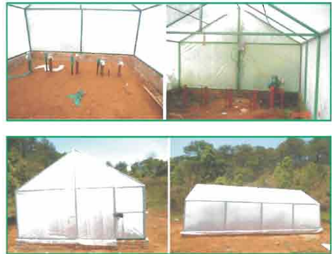
Fig 75. Poly tunnel with ETHE system
