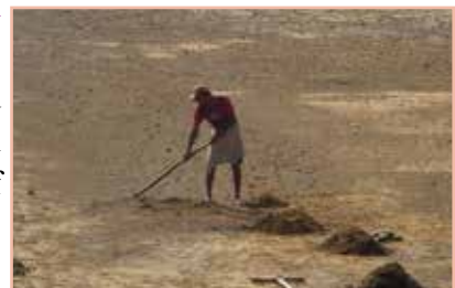
Scrapping of pond bottom
