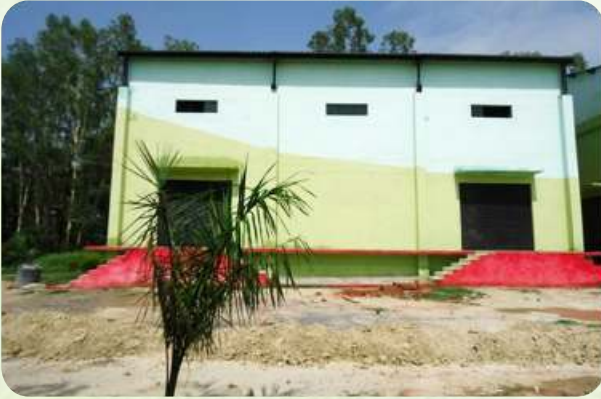
Seed Processing Plant
