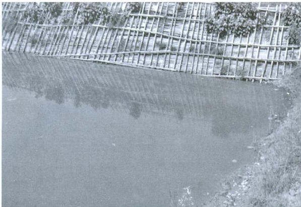
Fig. 3. Use of bamboo fencing for retention of pond dyke
