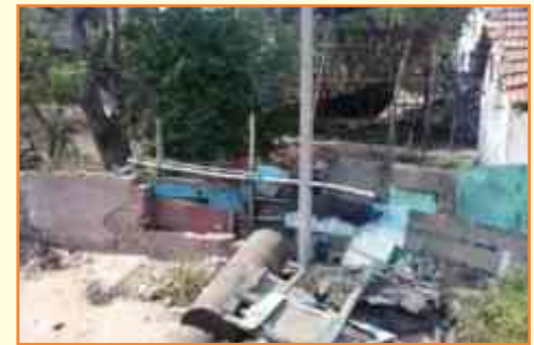
Destruction of residential houses due to disasters
