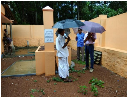
Open well renovated in the premises of Easanathukavu Devi Temple
