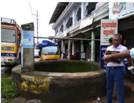
Open well in Vallapilly Market, Changanassery
