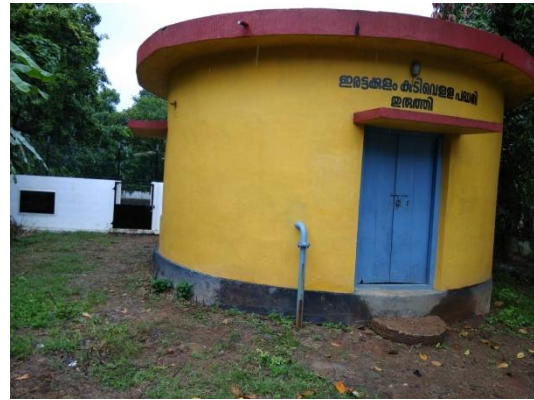
Open well & Pump House of Thuruthi Irattakulam Drinking water project
