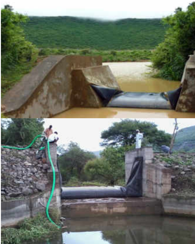
Fig. 3.1 Demonstration of inflation and deflation of the ICAR flexi check dam at Kanse village, Ambegaon Taluka, Pune district
