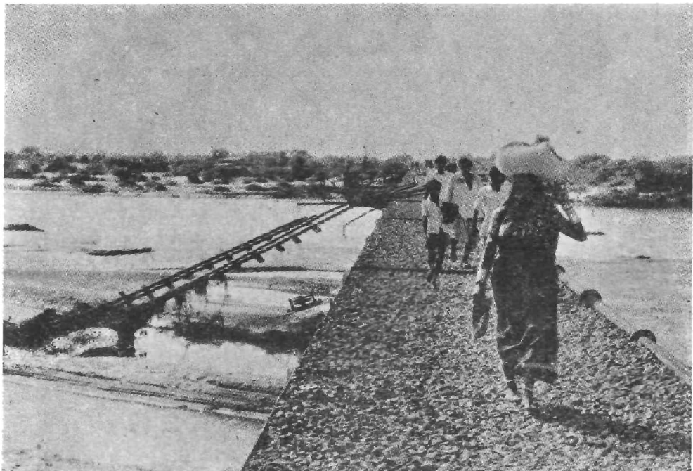
Scene over the railway bridge on the Luni. The track was washed away by the overflowing flood water.
