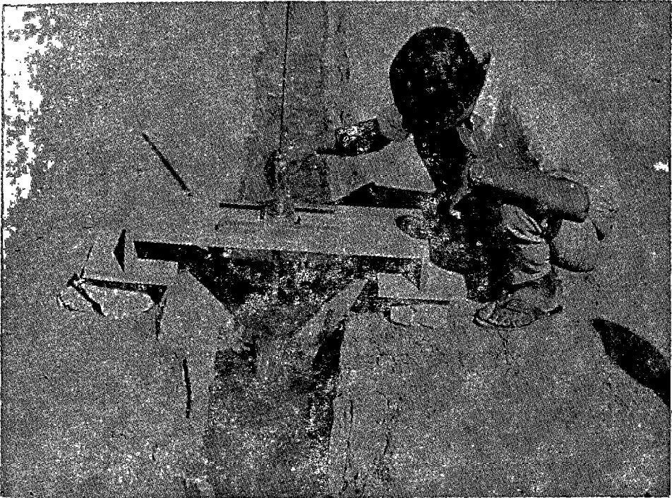
Measurement of flow in the unlined experimental channel.
