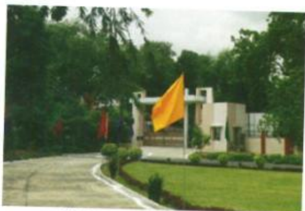
ZPD, Zone-IV, Kanpur office Campus
