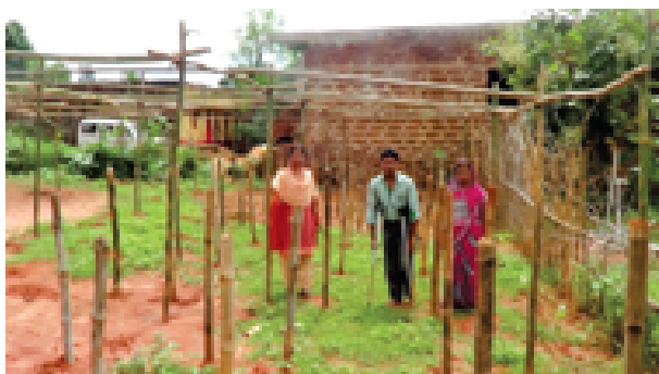
Constructing low cost bamboo structure for mushroom production
