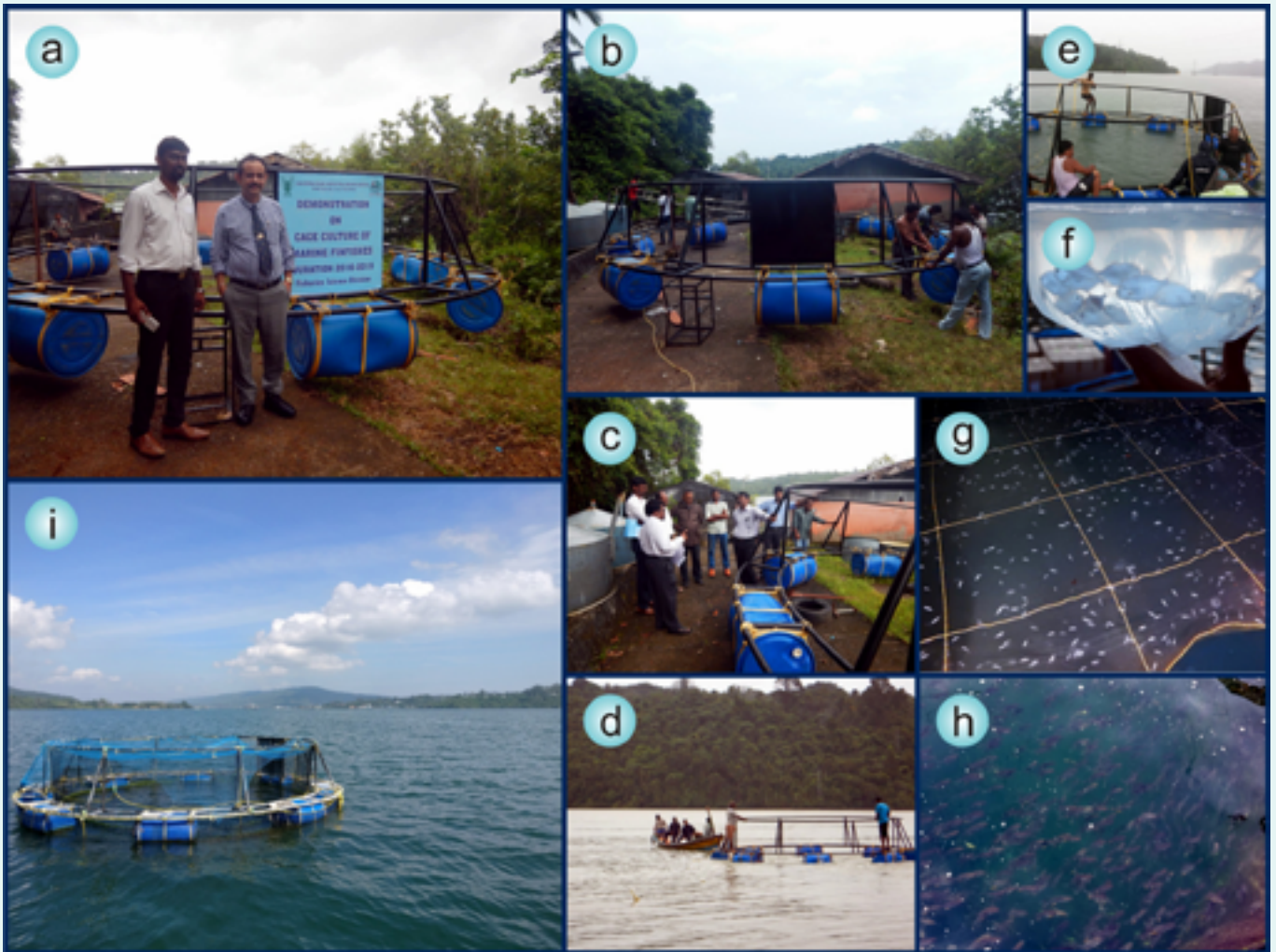
(Fig. 1) Construction of cage (a) and (b); verifying the construction of cage (c); transporting the cage frame to site (d); attaching the cage net and mooring the cage (e); stocking pompano seeds (f); pompano at 1 st day of culture in cage (g); pompano at 120 days of culture in cage (h); cage deployed at Minnie Bay (i).
