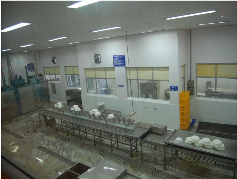
Fig: 03-Windows and ventilators
