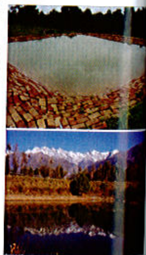
Plate : Poly-lined tanks for rain-water harvesting in hills
