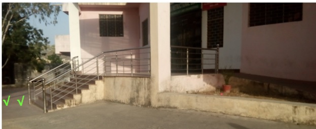
Fig 2: staircase along with to excess main entrance
