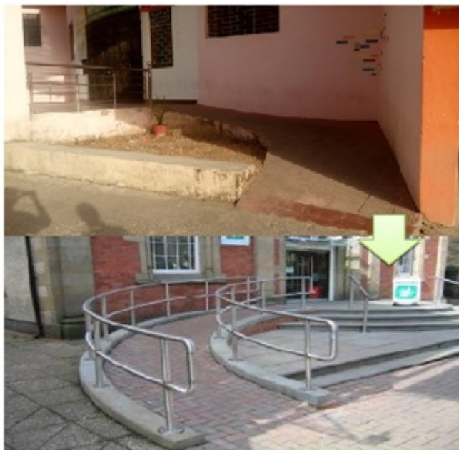
Fig 1: Ramp along with hand rails
