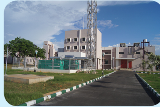
Standby power generation sets and Chiller of HVAC system
