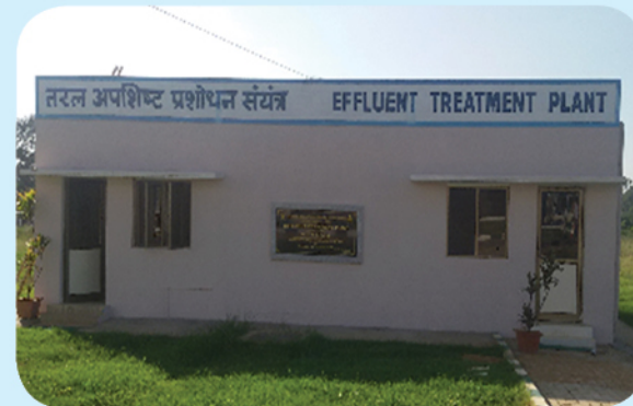
Effluent Treatment Plant
