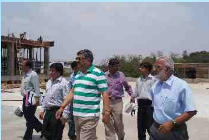
Dr. K.M.L. Pathak, DDG (AS), ICAR visited and reviewed the progress of the construction of Biosafety Laboratory and Administrative building of NIVEDI at Yelahanka, Bengaluru on 19 th April, 2014.
