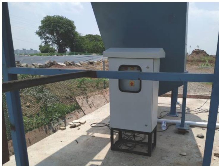
Water Filtration Unit
