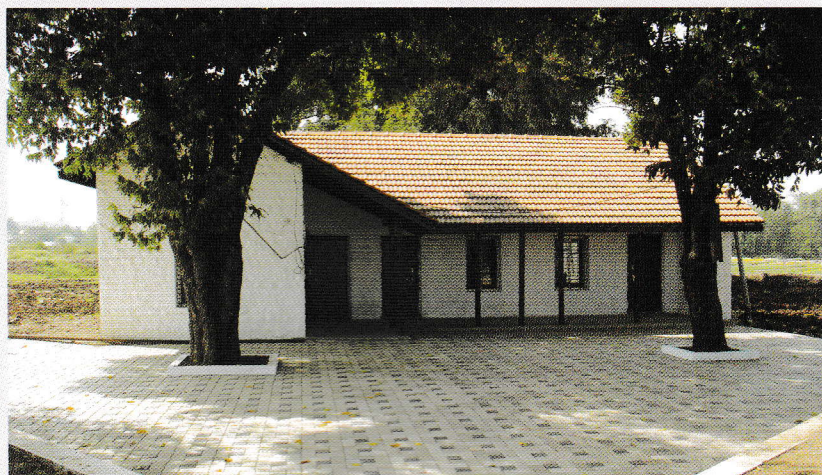
Renovated Transit office at Hadapsar farm of ICAR-DFR
