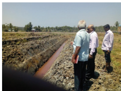
Drainage channels making
