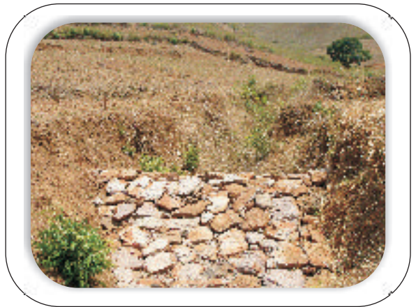
Gully control structure
