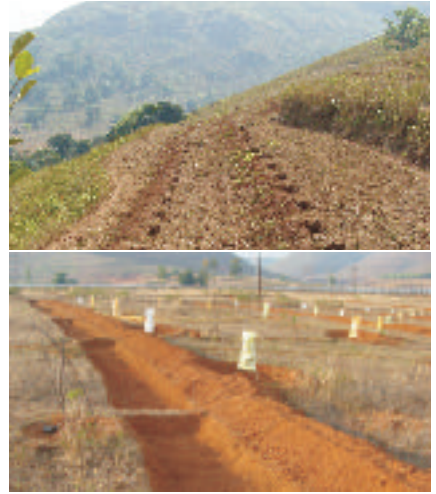
Photo 5.2: Trenching in non-arable land for rainwater harvesting
