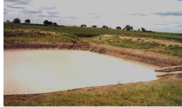
Photo 2. Farm pond at Joladarasi watershed showing inlet , outlet and spoil bank
