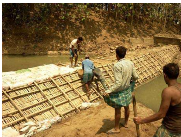
Fig. Rock fill dam construction: Converting the hazards into opportunities
