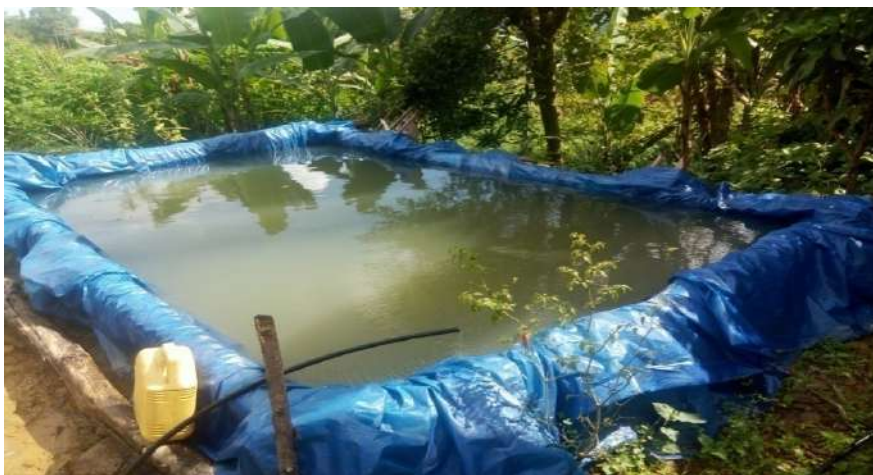
Fig. Jalkund for live saving irrigation
