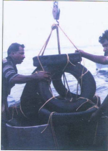
Fig. 1. Benthic FAD module, being deployed off Jodugullapalem, Visakhapatnam
