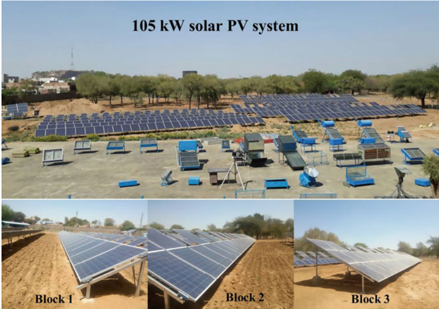
Fig. 6.3 Installed agri-voltaic system at ICAR-Central Arid Zone Research Institute, Jodhpur
