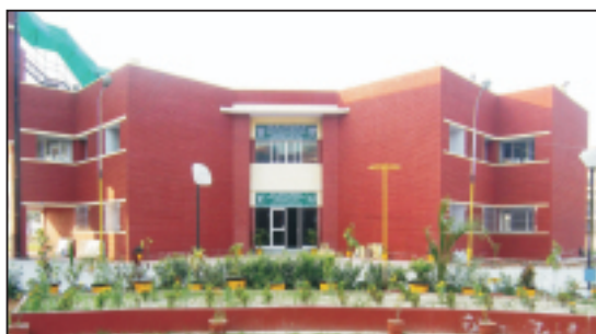
NBAIM new laboratory block
