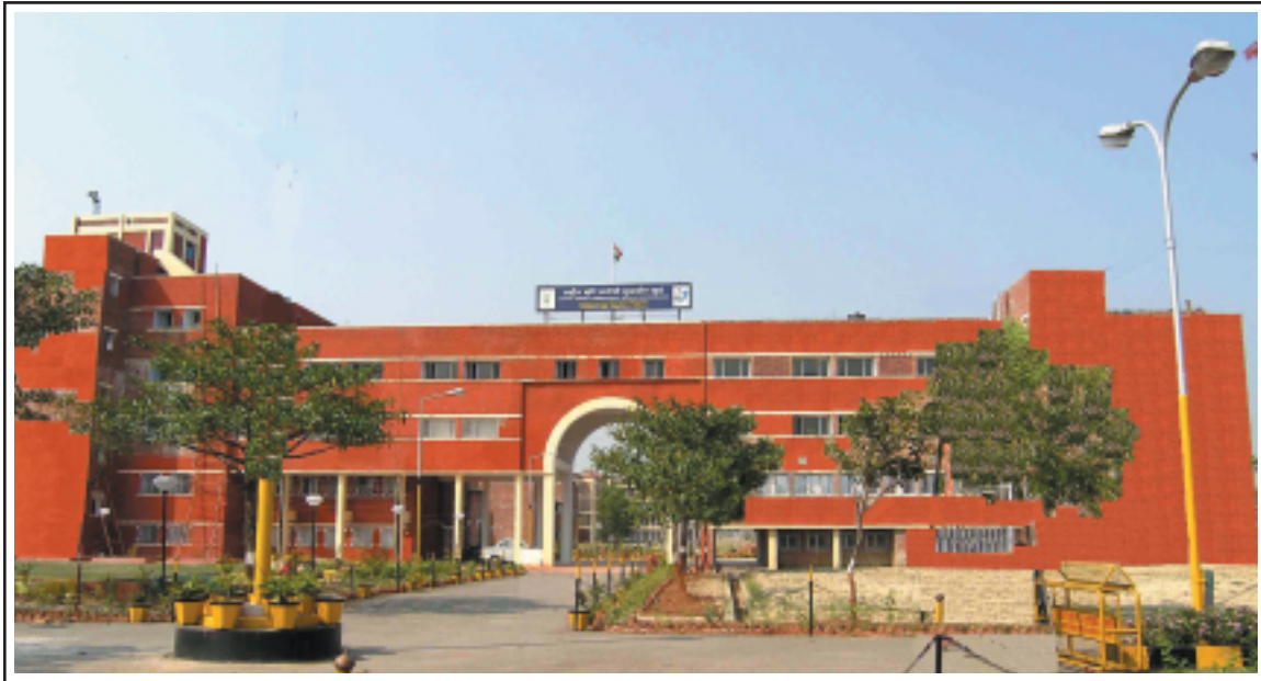
Front View of NBAIM & DSR
