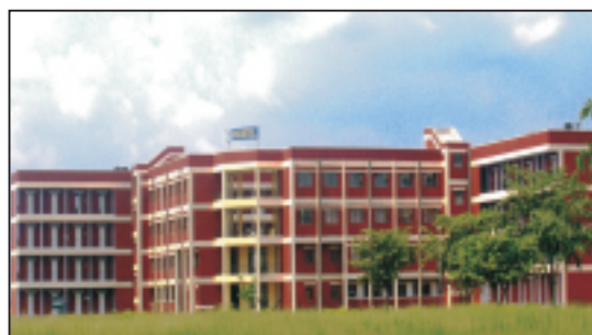
Far view of NBAIM / DSR Hostel
