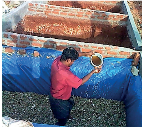
Figure 1. Silage pits lined with plastic sheet to prevent seepage.
