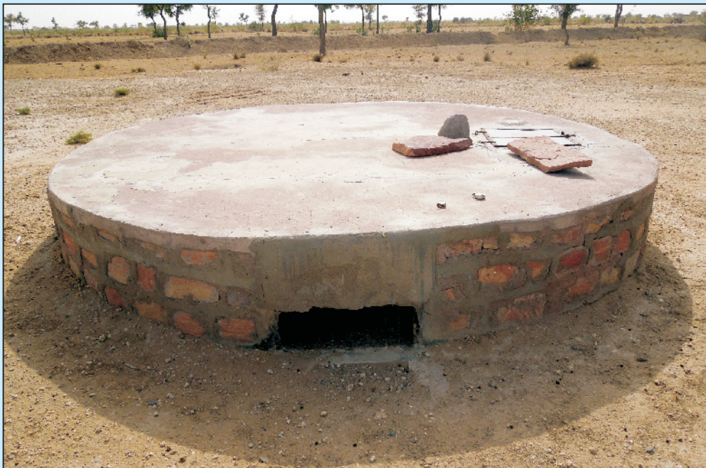
Tanka constructed under watershed program
