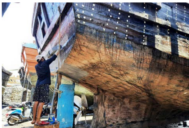
Fig. 3 Application of paint
