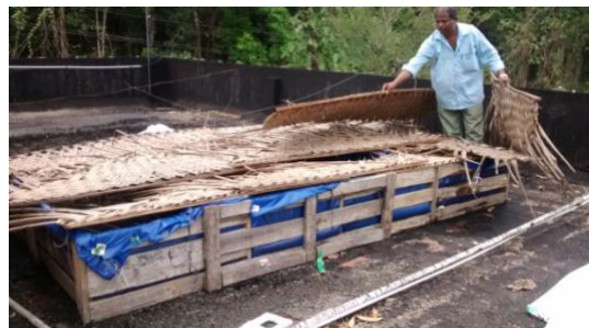
Pools setup on rooftop using wooden planks and siplaulin sheet
