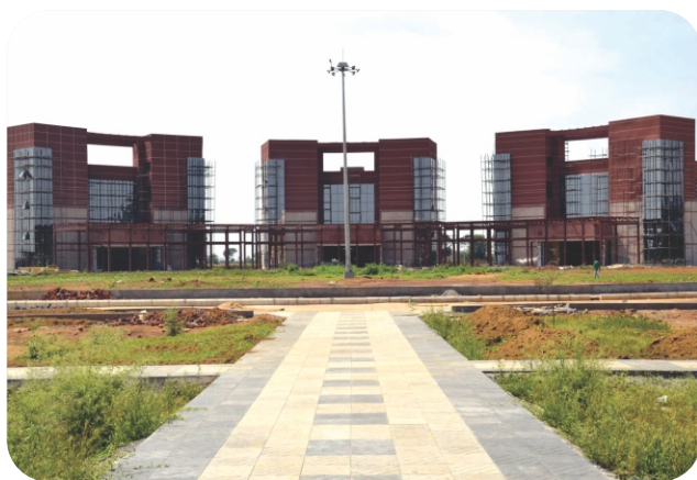
From left Auditorium, Admin and Library
