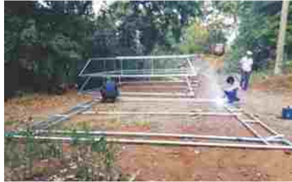
G.I. pipes welding for cage frame
