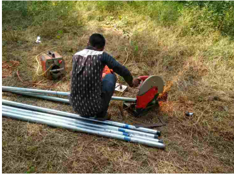
Cutting of G.I. pipes for making frame
