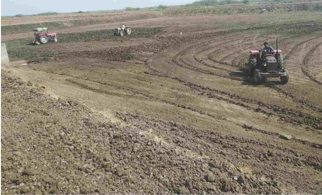
Ploughing of pond bottom soil
