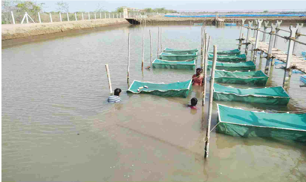
Bamboo installation and hapa fixation
