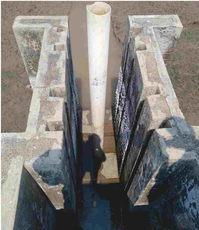
Sluice gate structure
