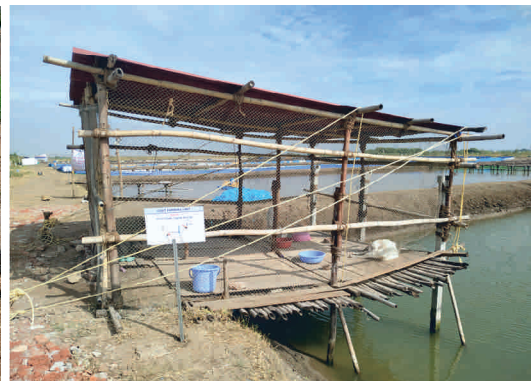
Low cost goat rearing shed on pond dyke
