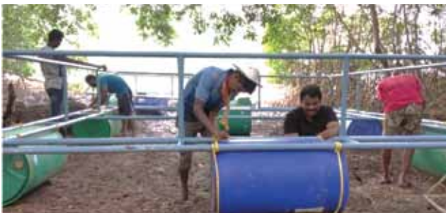
Barrels fixing and cage frame installation by SHG members
