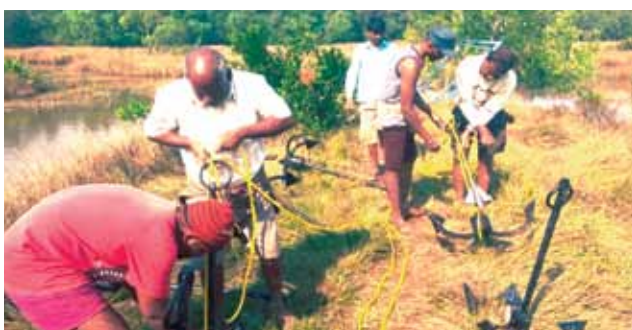
Anchoring cage frames
