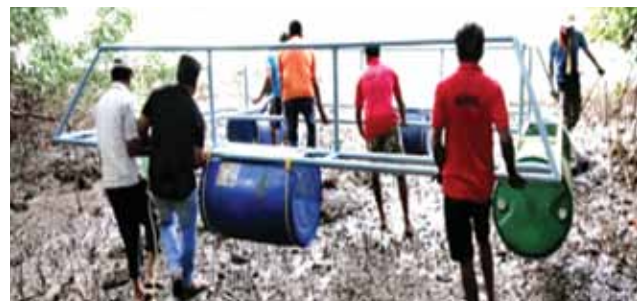
Barrels fixing and cage frame installation by SHG members
