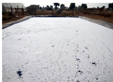
Water storage pond with surface covered with thermocol balls
