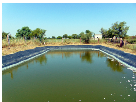
Water storage pond without thermocol ball
