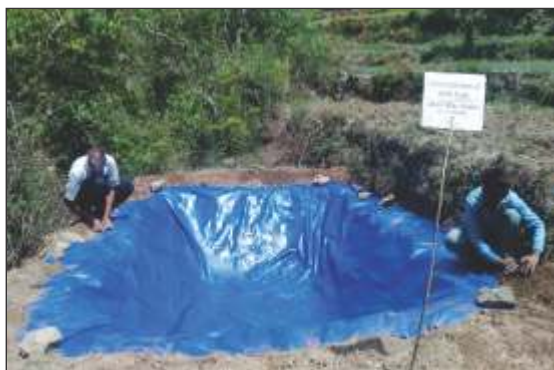
Construction of LDPE tanks at village Bharkote in Uttarkashi
