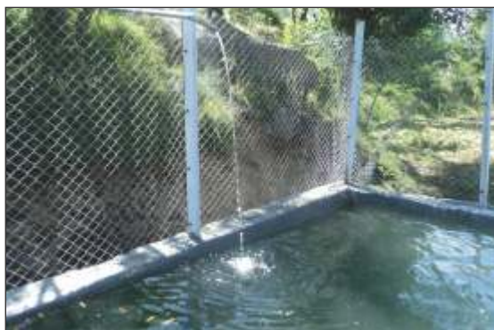
Water storage structures
