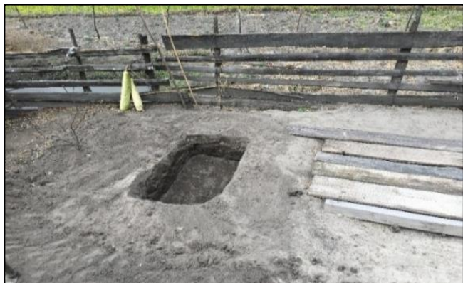
Fig 1: Digging of pit
