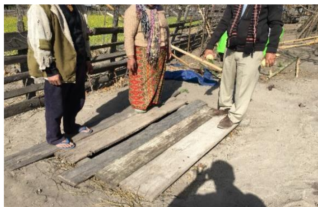
Fig 8: Last covering the pit with the wooden planks layer
