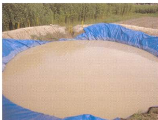
Photo 4b, After rainwater harvesting upto 60,000 litre, this micro pond with a raised embankment (4.0') of dug out soil, can retain 1,00,000 lit of water (lined with 42 ' X 42' size sipaulin sheet), if it is filled up by pump from standing water available in the field itself during heavy rain to sustain jute retting and jute-rice-rabi cropping sequence.
