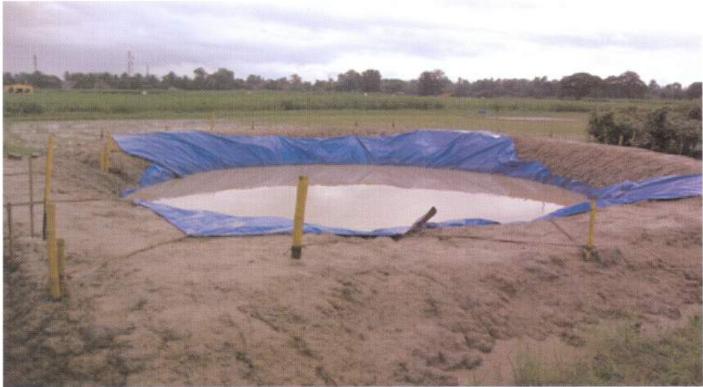
Photo 26. Rain water harvesting with higher storage (1 lakh litre) using dug out soil for jute retting and sustain jute –rice –rabi crops in sequence.
