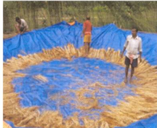
Photo 3. Micro pond and its lining with silpaulin/polyethylene sheet and circular straw bed as cushion material along the bottom periphery for insitu jute retting using ground water.
