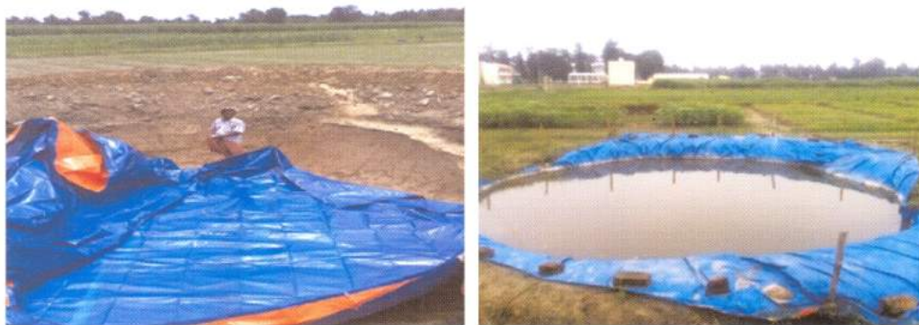
Photo 4a. Micro pond for insitu jute retting using collected runoff water from jute field (60, 000 lit approx.)
